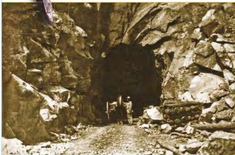
East portal of summit tunnel of the Central Pacific Railroad, during construction in the Sierra Nevada Mountains, California.
