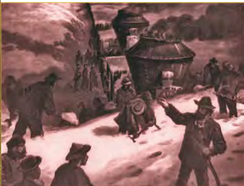
Snow didn't stop work on the railroad. Here, Chinese laborers dig a train out of a drift near Ogden, Utah.
